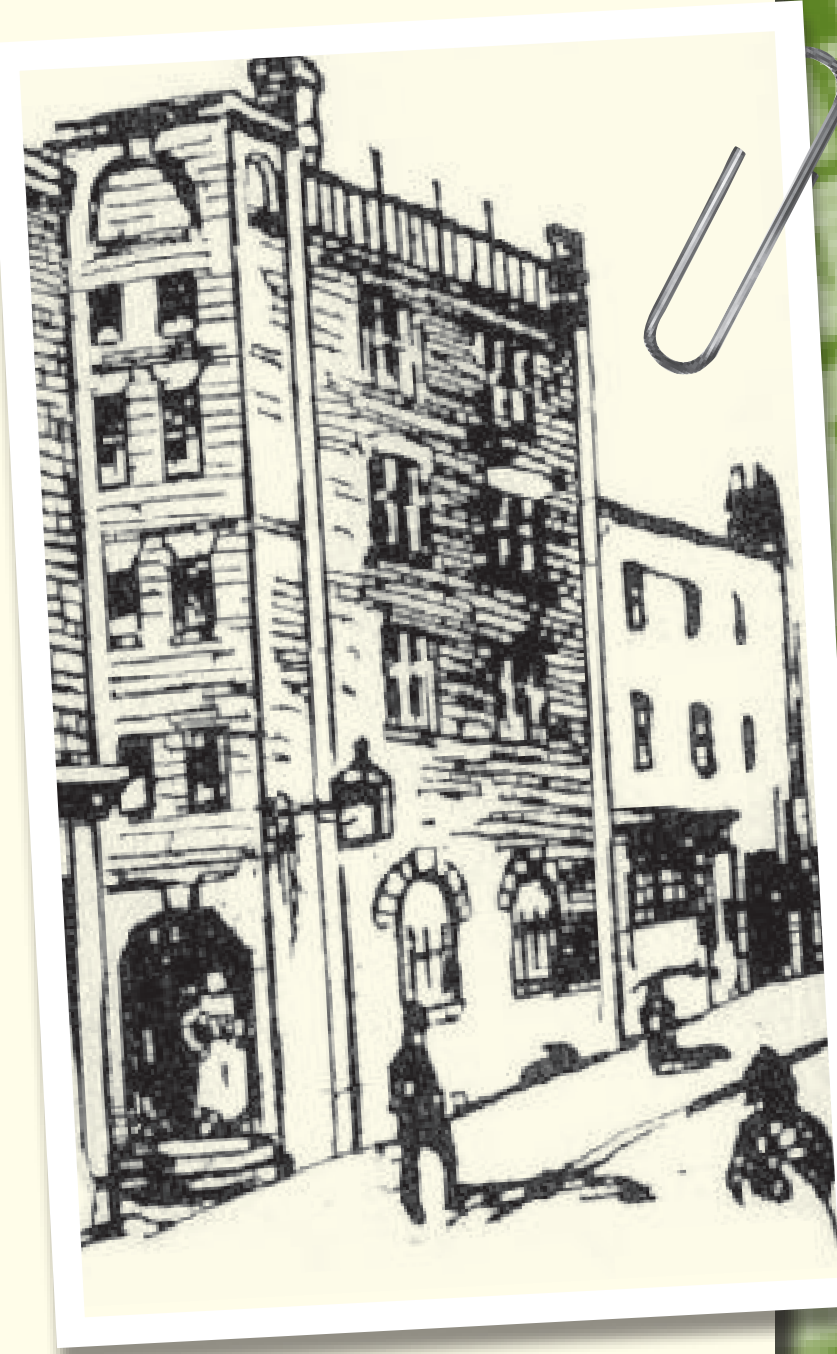
ENTRANCE TO MILLER'S COURT
